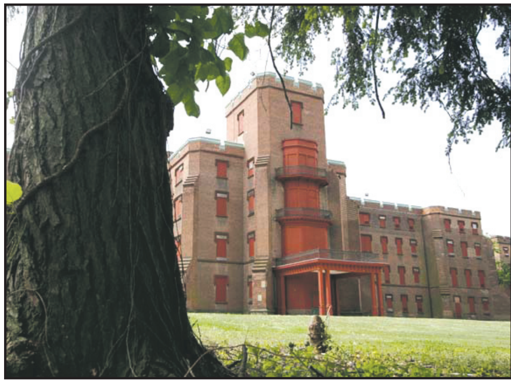
BY LINDA DAVIDSON — THE WASHINGTON POST The Center Building at St. Elizabeths would be renovated and become part of the federal Homeland Security Department complex. The $3.4 billion headquarters would provide a workplace for 14,000 federal employees.
